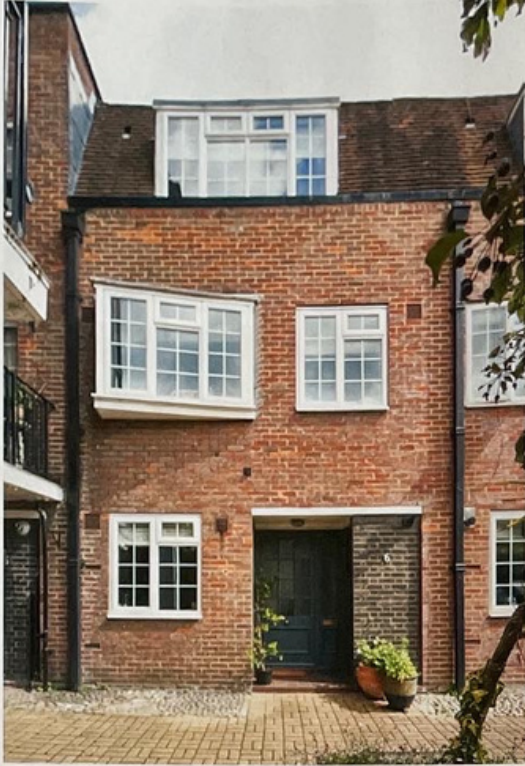
ABOVE A 1970s-build has been updated with a front door painted in a modern neutral. BELOW A trio of townhouses by Squire & Partners echoes the symmetry and scale found in surrounding Victorian properties.
