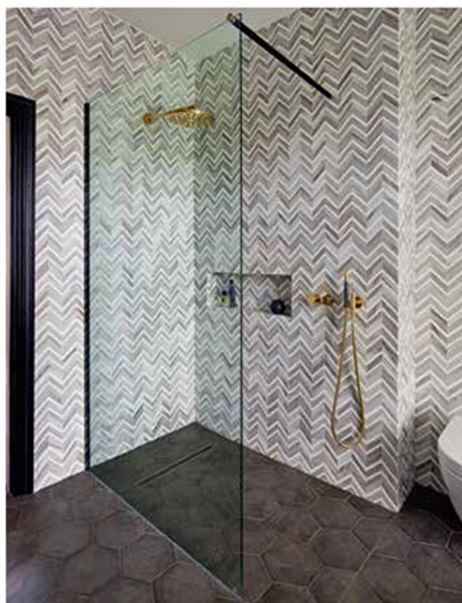
ABOVE A frameless screen helps to achieve a luxurious wet-room appearance and allows the tiles to come to the fore, with a neat niche for toiletries contributing to the elegant minimalism of the scheme.
